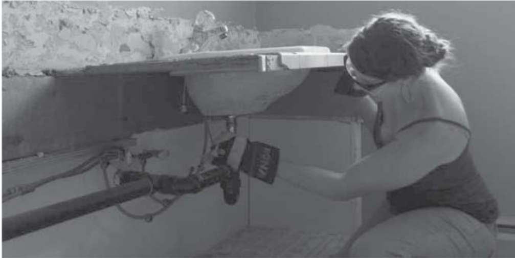
Kristi Hansen is a Red Seal plumber. Calculating the capacity of water lines, determining the length of pipe needed for drainage systems, and accurately predicting the volume of hot water a building's system will use are some of her tasks.
