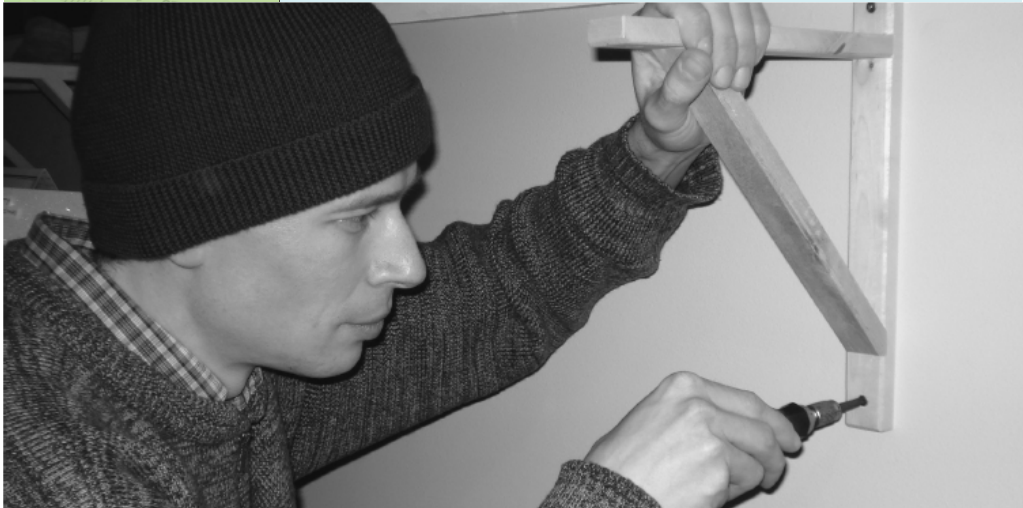
This man is installing an angle brace. By incorporating right triangles, angle braces provide support and strength to bookshelves, building roofs, and beyond.
